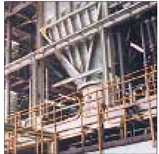
RockShield 60 has excellent wear characteristics in chutes, hoppers, bins and transfer points.
